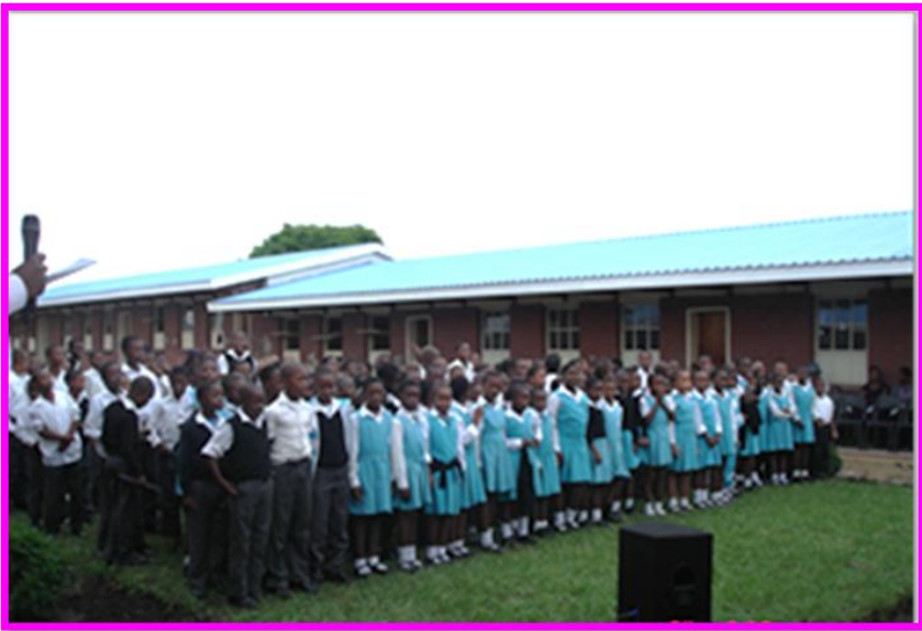
2012JFY: Construction of Library in Imfanelo S. P. School, Uthukela (R599,497)
