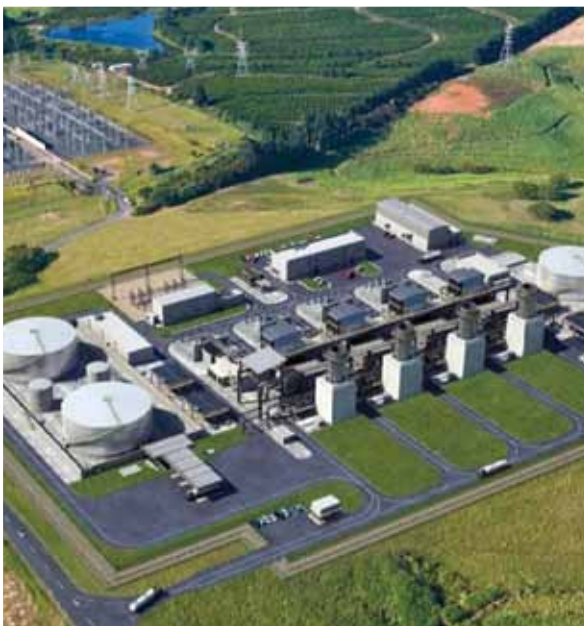
Image photo of the Avon Peaking Power Plant
